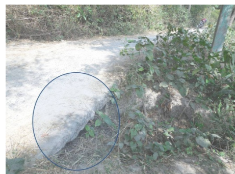
Photograph of one point of gap between the surface and the road in Balarampur road, Baliapal
