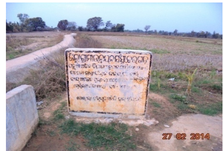
View of canal embankment constructed out of CC Road funds at Karandola, Sohela PS
