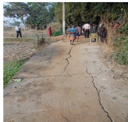
View of the cracked road at Balabhadrapur, KM sahi, Jaleswar
