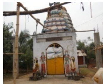
View of newly constructed temple at Tangi-Choudwar Block
