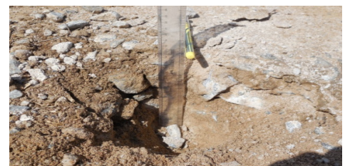
View of measurement taken on a cracked road at Majurai, Jharapada in Kantapada PS where the chips layer was 1”
