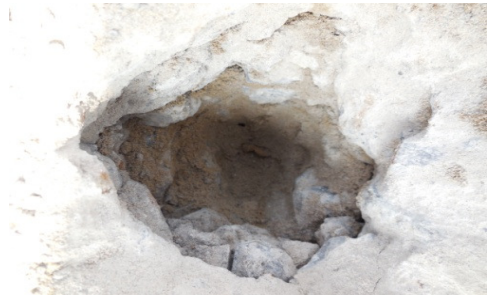
View of the hole made on the road at Kudumansingh, Baliapal PS exhibiting absence of metal layer
