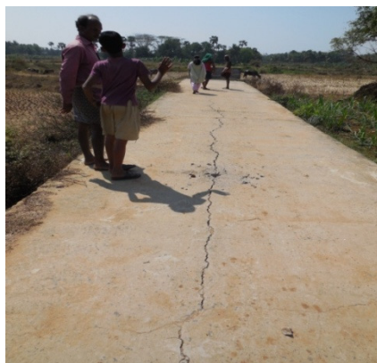
View of a cracked road at Bhakarkuda, Olatpur, Kantapada PS
